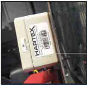
Hartex Panel Alarm installation for Fire Suppression System
